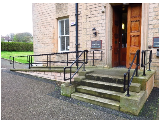
Access ramp photo
