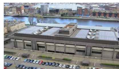
Solar Panels on the roof of Glasgow Sheriff Court
